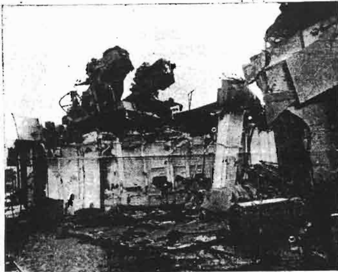
DAMAGE ON RAMMED DESTROYER.—Picture shows damage done to deck structure of US destroyer Charles H. Roan when the destroyer Brownson collided with her in manoeuvres last Wednesday. Centre left is the first of the two after gunmounts into which the Brownson's bow rammed after demolishing quarters on deck. Not shown in picture is gaping hole torn in starboard side of Roan's hull.
